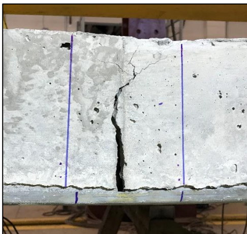
(a) Fissura principal
