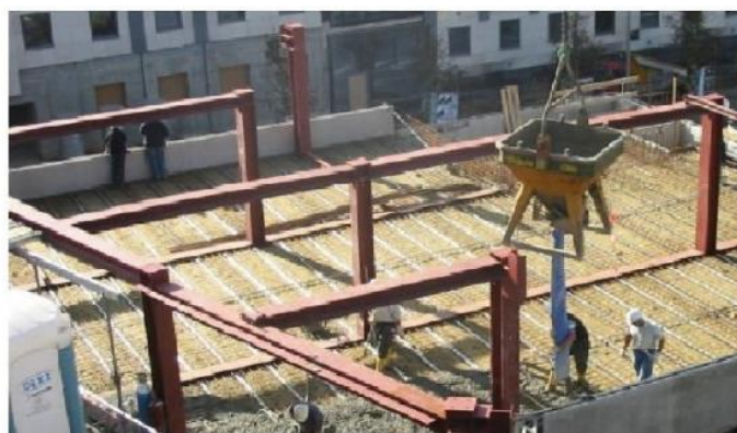
(b) ArcelorMittal Office Building Petrusse
