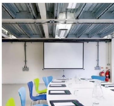
(c) The Boilerhouse
