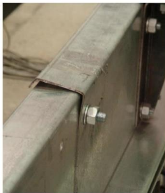
(b) Falha distorcional.
