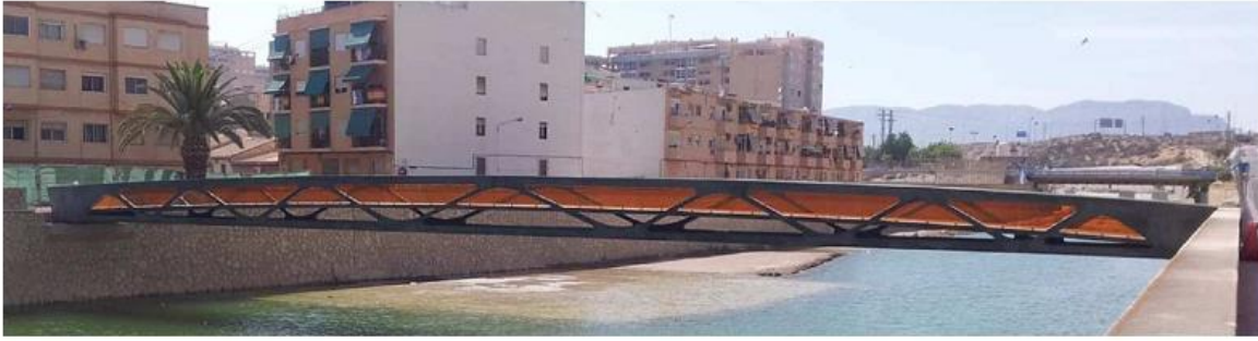
Figure 1 – UHPFRC pedestrian bridge over the Ovejas Ravine, Alicante
