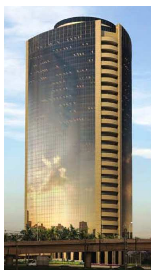
(a) Edifício Tower Bridge Corporate (SPCORPORATE, 2012)
