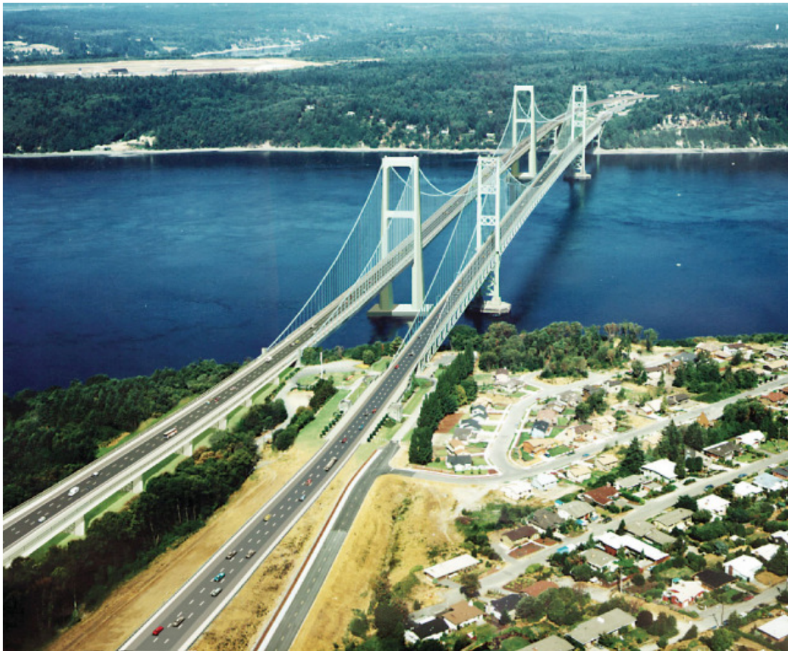
Figura 1.4 - Nova Ponte Tacoma Narrows, Jones e Treyger (2005)
