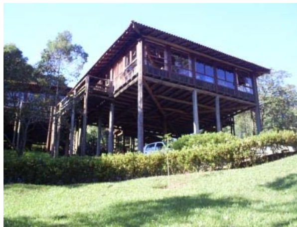
Vista do Pavilhão Don Duane Willians (10mx10m).
