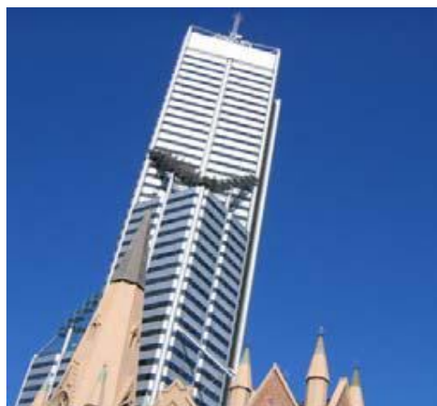
d) Central Park Tower – Perth, Austrália
