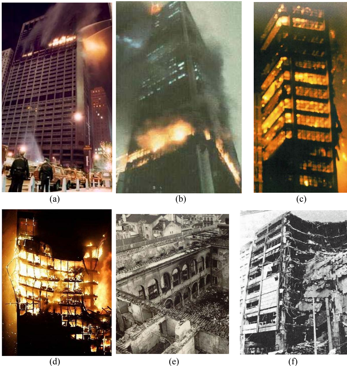
Figura 2.14 - (a) Meridian Plaza na Filadélfia - EUA, em 1991, (b) Edifício do Firts Interstate Bank em 1988; (c) Edifício da CESP, em São Paulo — 1987; (d) Torre Windsor, Madrid, 2005, (e) Museu Colonial de Lisboa; (f) Edifício Katrantzos Sport, em Atenas, na Grécia — 1987; fontes (a) http://911research.wtc7.net/talks/b7/history.html , (b) http://911research.wtc7.net/cache/wtc/analysis/compare/lafire_firstinterstate.htm , (c) e (d) http://www.lmc.ep.usp.br/people/valdir/?page_id=16 , (e) http://www.triplov.com/politecnica/fotos_museu_bocage/pages/a_incendio.htm e (f) http://www.fpemag.com/archives/article.asp?issue_id=27&i=153 .
