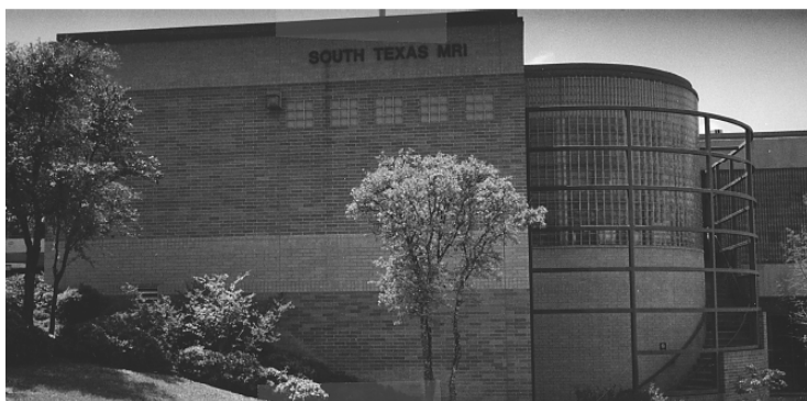
Figura 1.2 – Hospital no Texas (ACI 440 R, 1996)
