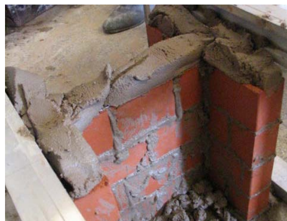
d) Argamassa cobrindo as telas
