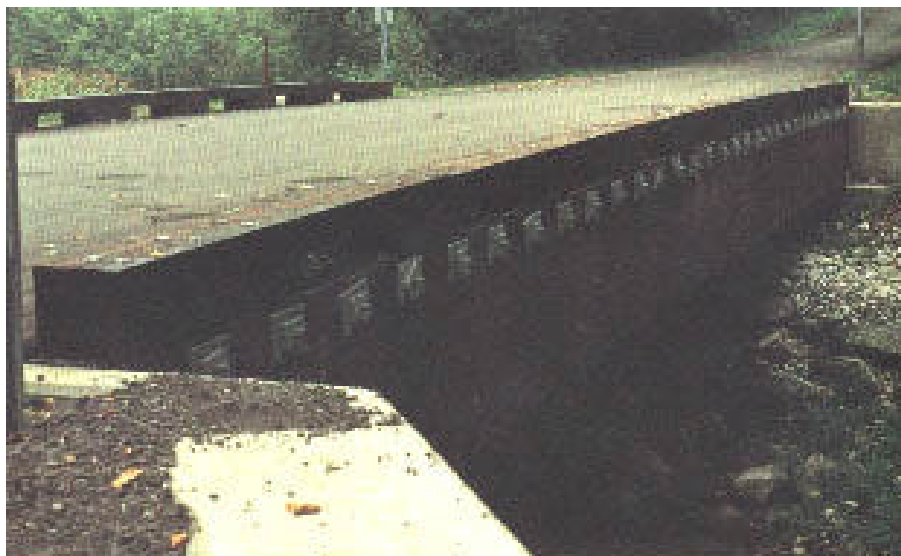
FIGURA 20 - Ponte "Camp Arrowhead" (USDA Forest Service, 1995)
