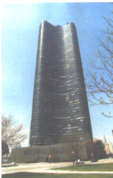
Figura 1.2 - Lake Point Tower, Chicago [GONZALEZ-ISABEL(1993)]
